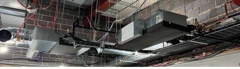
which was connected, thermally insulated, and balanced onto linear grilles was installed the full length of the office space. Hybrid systems utilise part refrigerant / part hydraulic water, therefore requiring a category 5 break tank, PRV, pressure monitoring and distribution pipe work to the HVRF selector box for filling of the hydraulic water circuits of the system.
